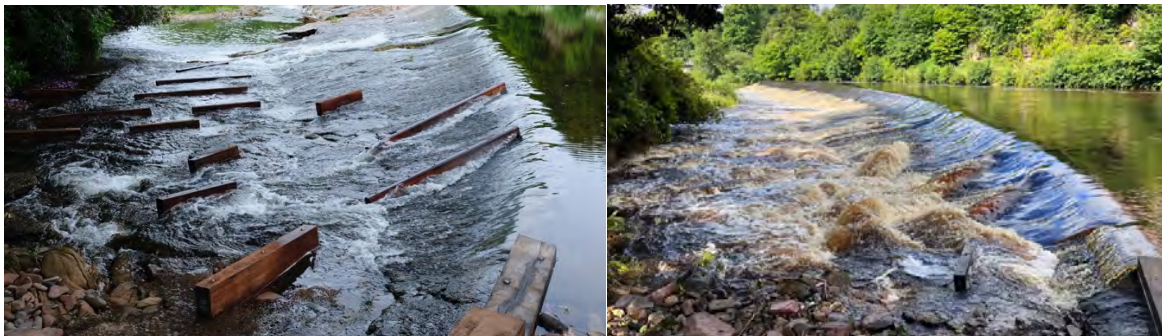
Sorn Castle Dam baffles in low flow on the left and in a small spate on the right. This will make fish passage easier and poaching harder
