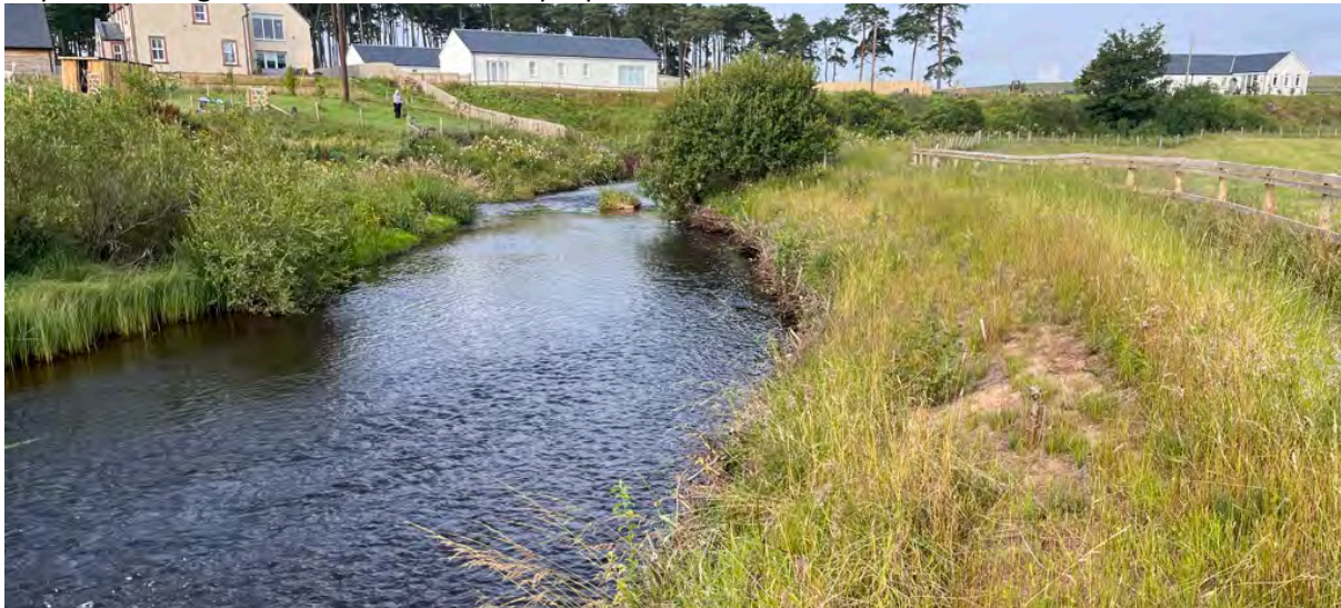
Nether Wellwood has benefitted from two bank stabilisation installations recently
