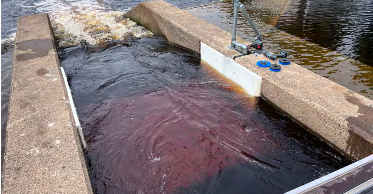
The counter within the upper fish pass at Nethermills after a weekly clean
