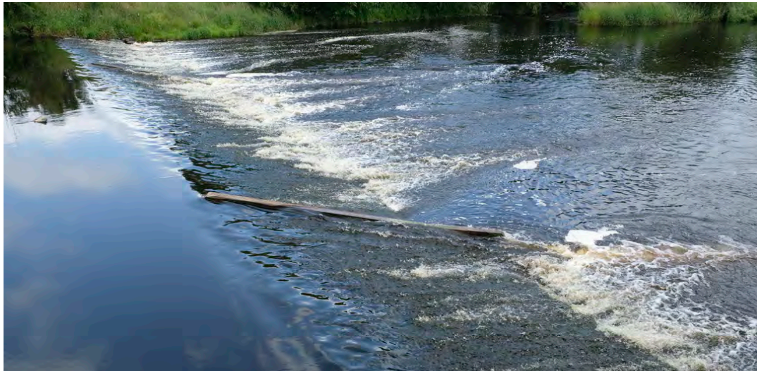
Two 6m timber baulks added to help salmon and trout migrate over the dam in low flows
